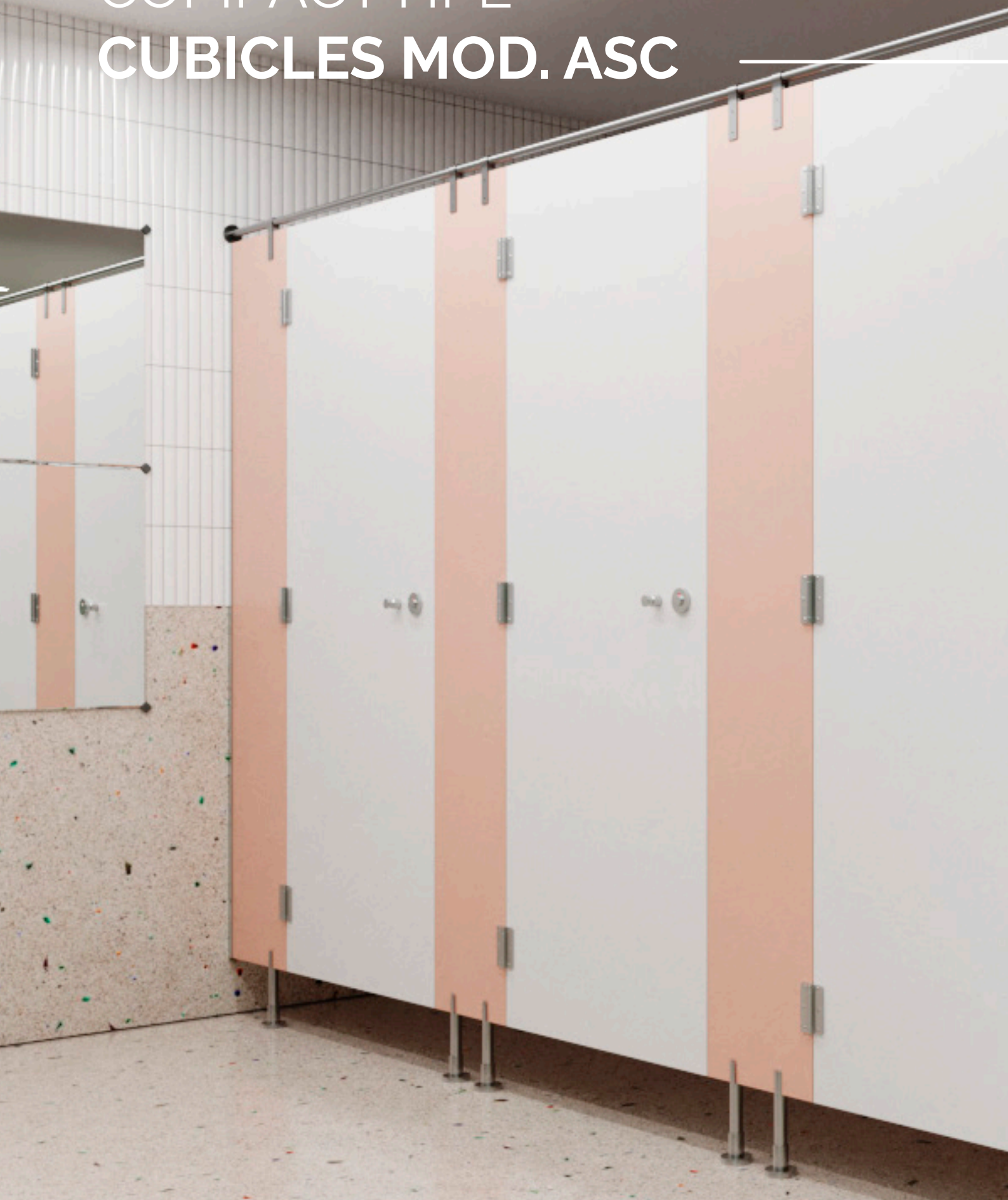
Toilet and shower cubicles.
